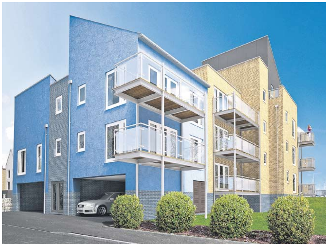
St Mary's Island: The new development was saved by £7m Kickstart funding Creditm to come
